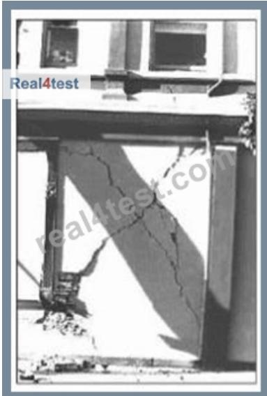
Refer to the exhibit (photo showing diagonal cracks in a wall).
